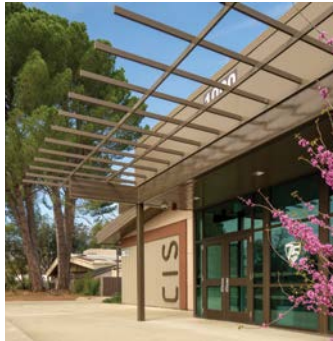
Computer Information Systems (CIS) Building October 2021
