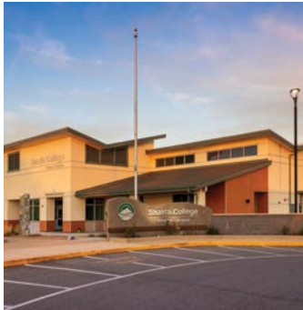
Tehama Student Services Building November 2020
