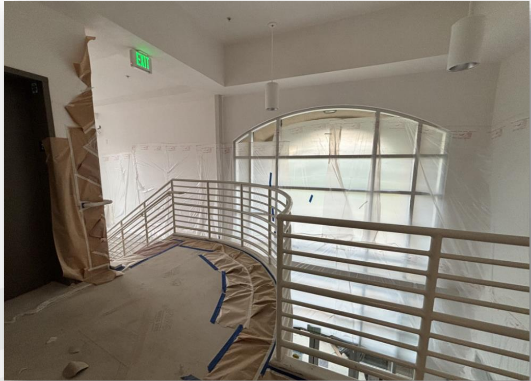
Handrail Painting Prep
