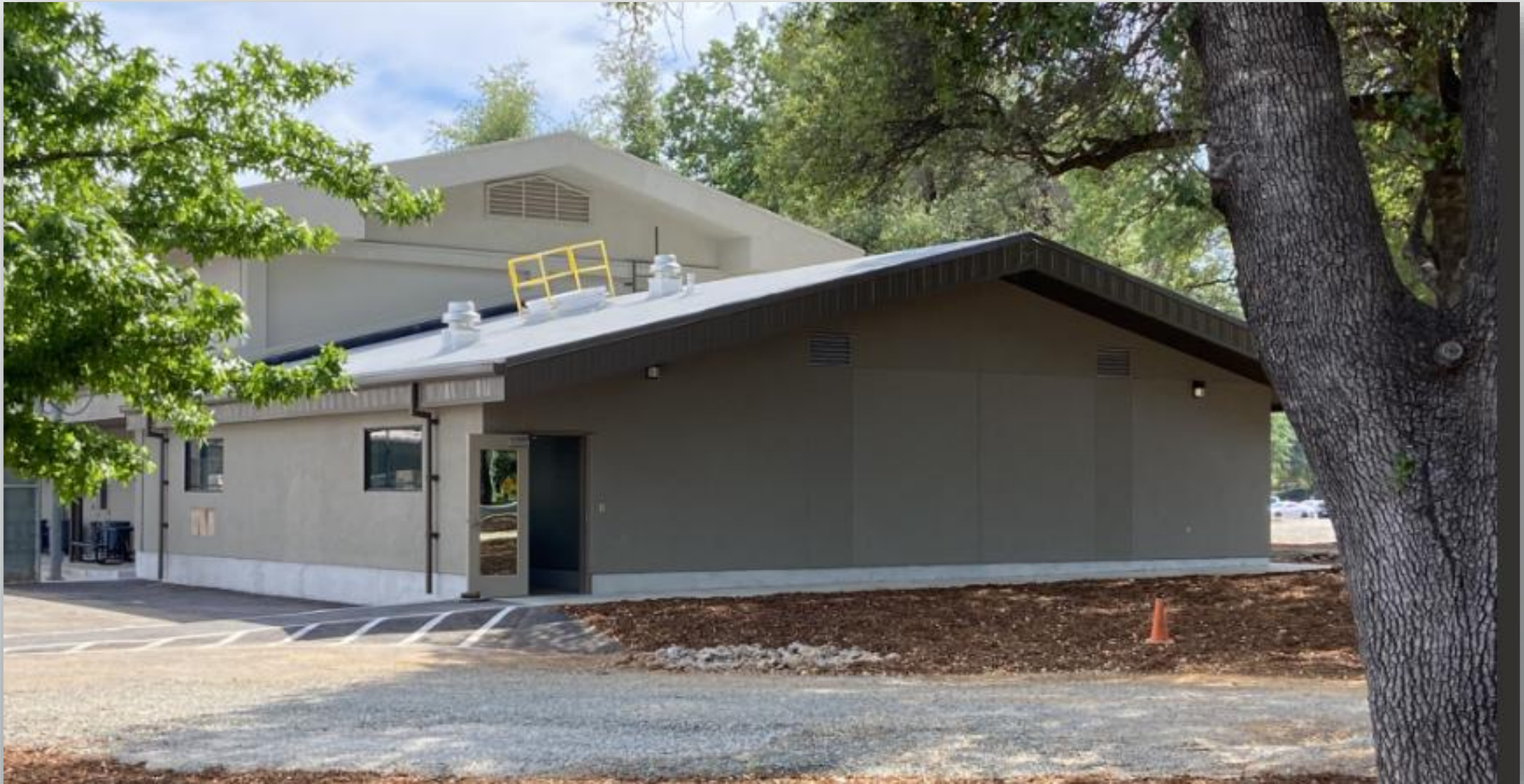
CAL FIRE Redding Training Center Cadet Housing & Locker Rooms
