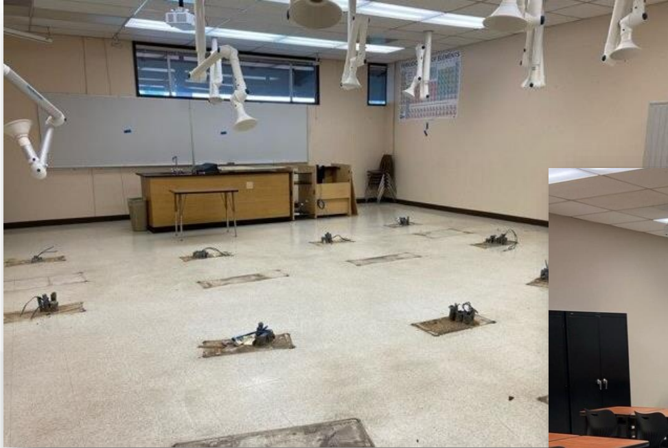
Room 1411 Before & After
