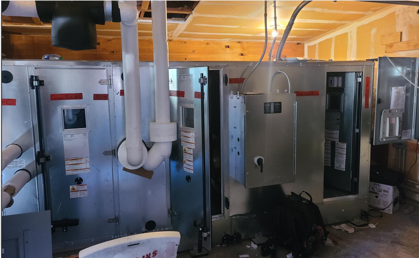
Air Handling Units above the Cafeteria kitchen area
