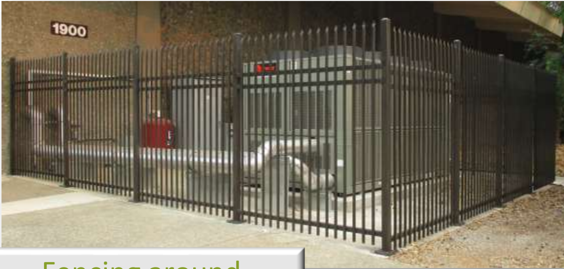
Fencing around equipment on the west side of the 1900 Building (Gym)
