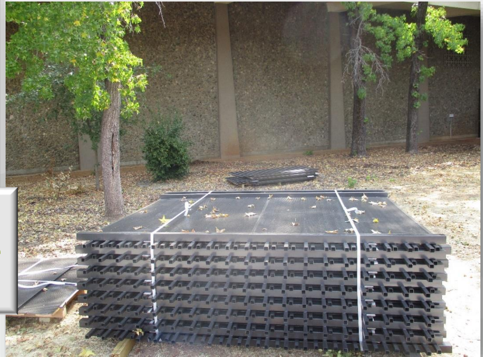
Fencing for equipment on the west side of the 1900 Building (Gym)
