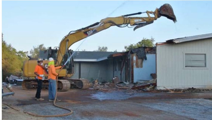
DOJ Building demolition
