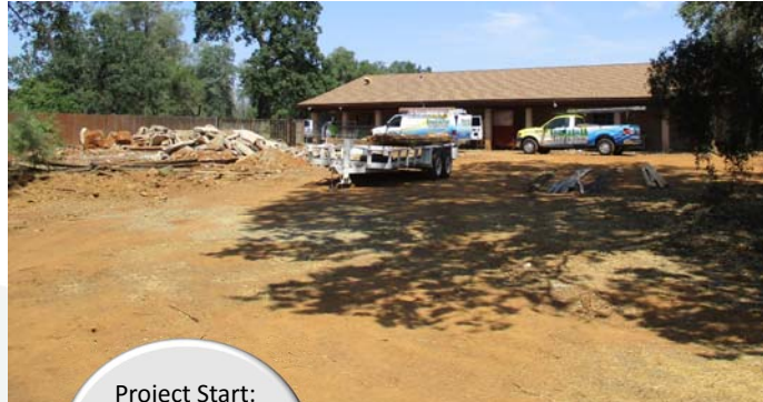
Area cleared behind the Campus Safety Building (Bldg. 6500 - under renovation)
