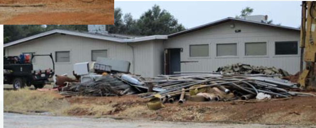
Excavation and Demolition
