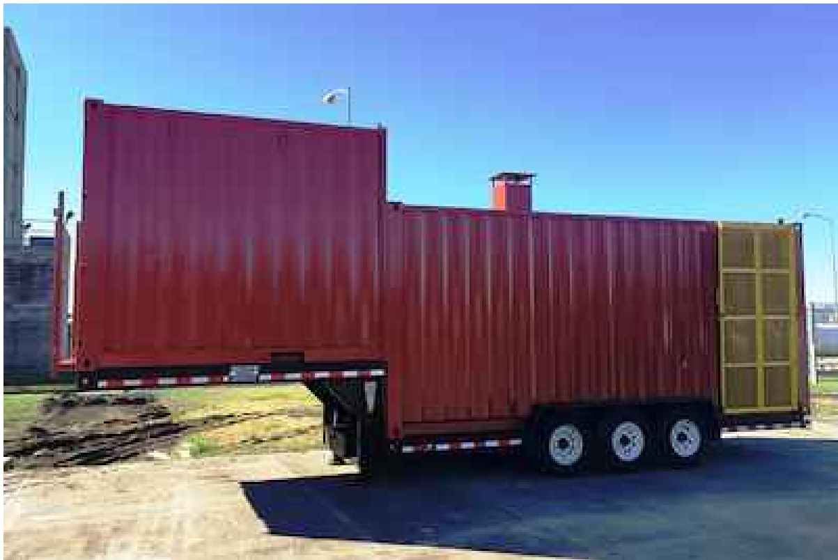
Dräger Survival System Phase I – Flashover Development Observation Burn Building
